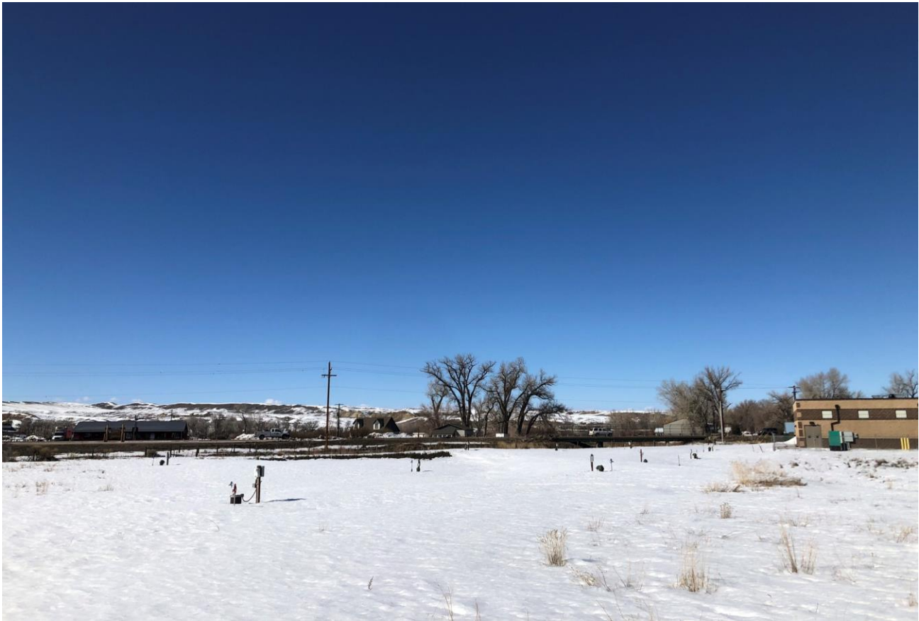
Alluvial Wellfield and Treatment Plant
