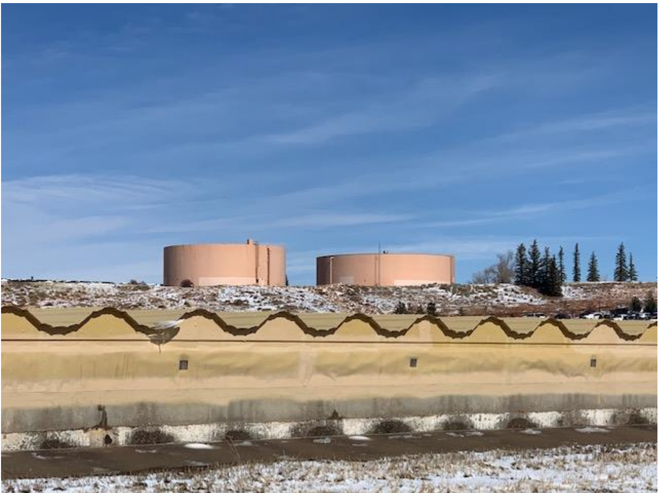
Zone 2 water storage tanks (capacity: 2.1 million gallons and 1.5 million gallons)
