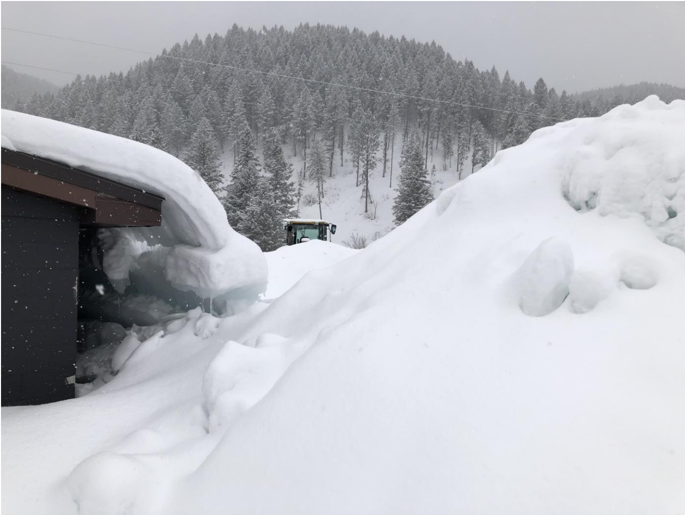
Control Building Roof with Snow
