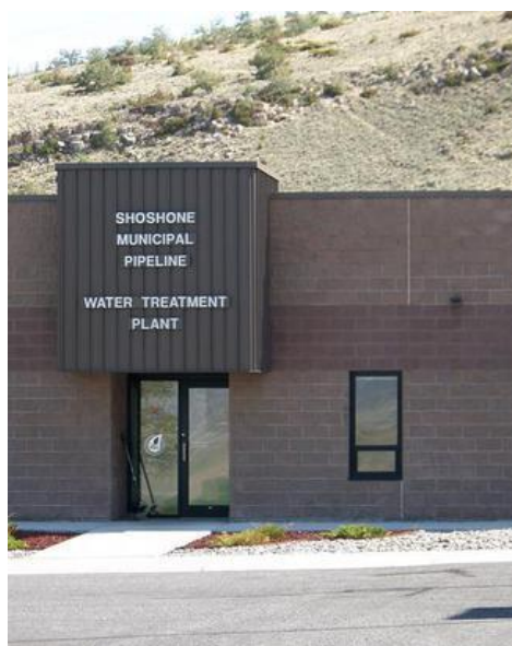
SMP Water Treatment Plant
