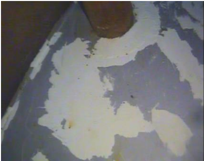
Interior Floor Patching
