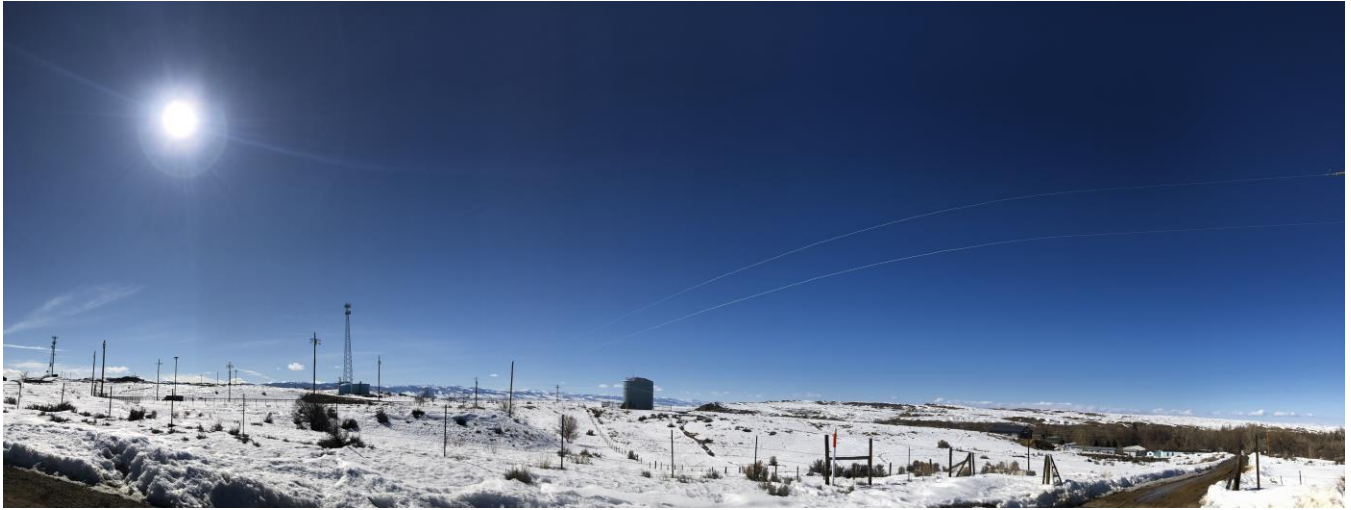
Storage Tanks for Potable System and Cemetery Landscaping
