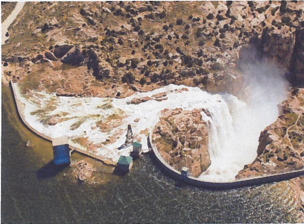
PATHFINDER DAM SPILLWAY - 2010
