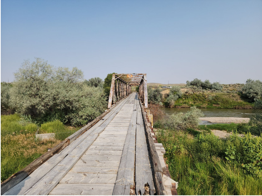
Overall Picture of the Flume
