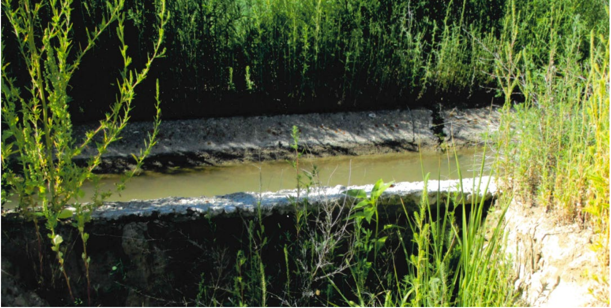
Concrete Ditch Portion of D44-10
