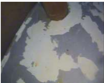
Interior Floor Patching
