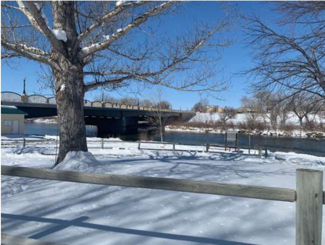
One of the two river water main line crossings on the North Platte River, west side of the City of Douglas.
