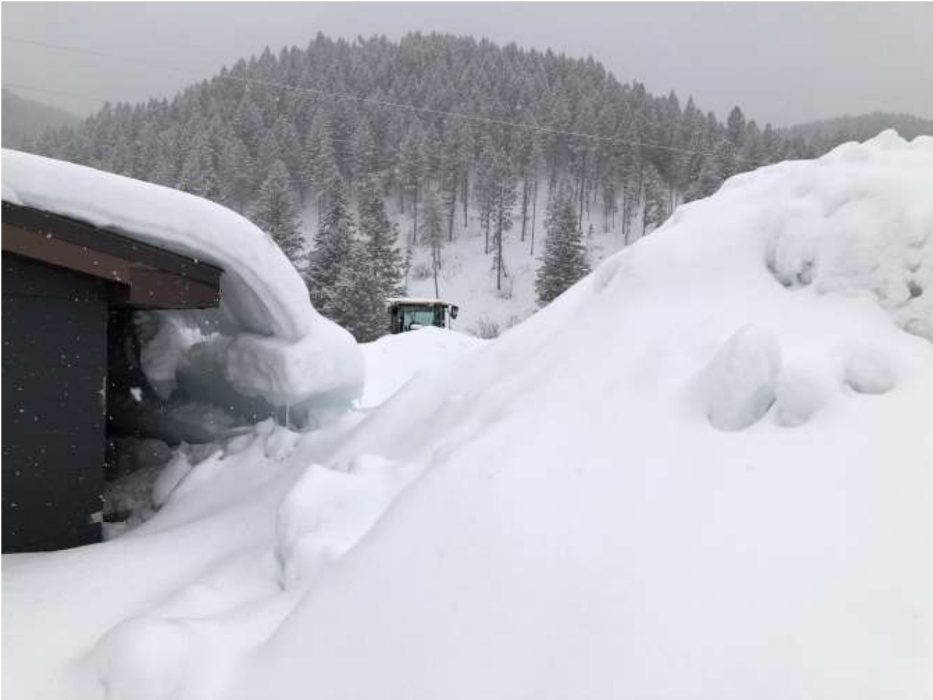
Control Building Roof with Snow
