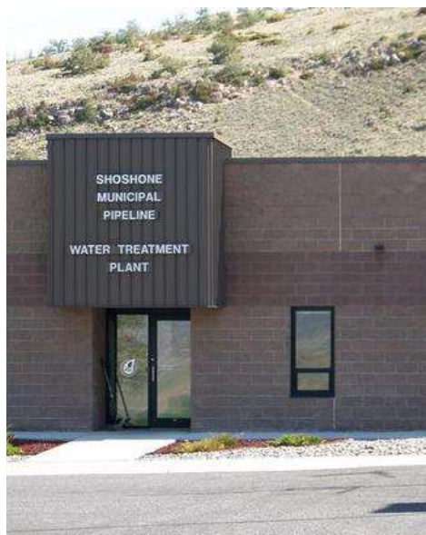
SMP Water Treatment Plant
