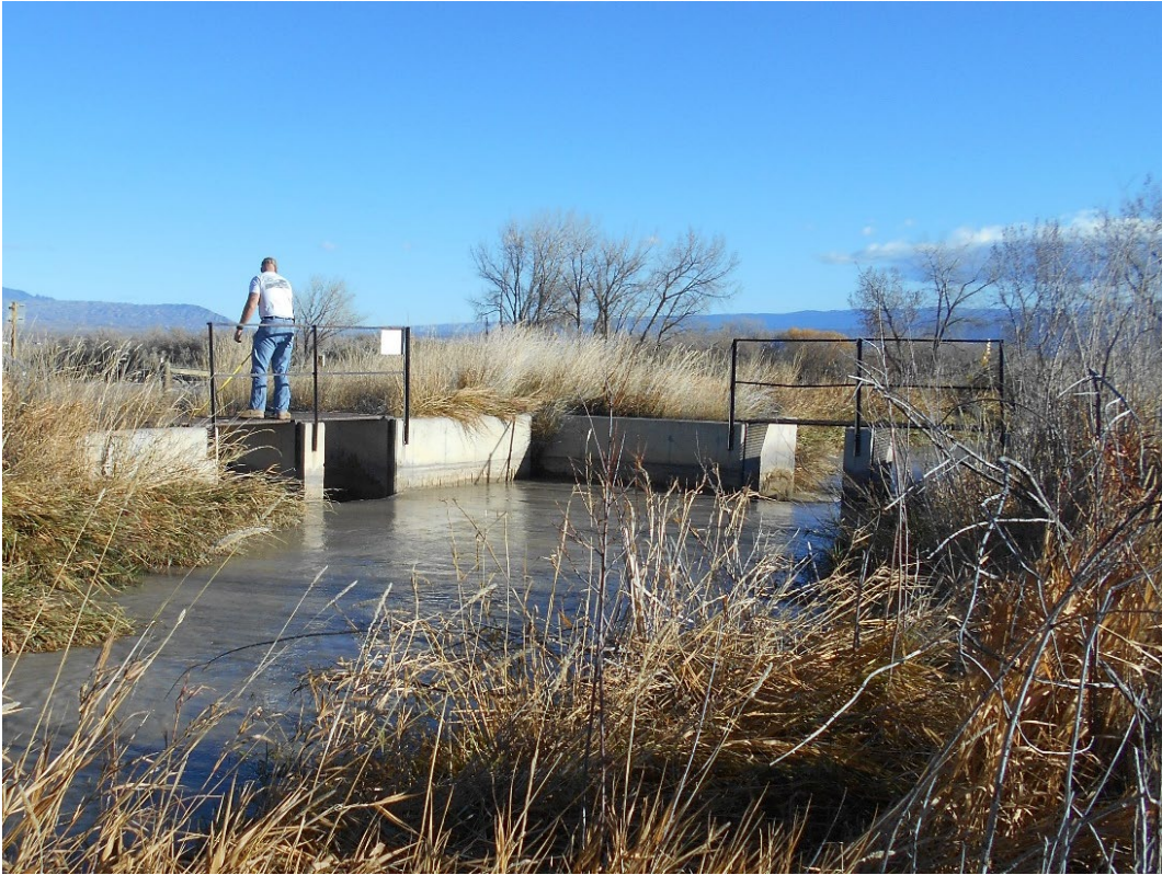
BENCH DIVERSION - BENCH STOP LOG WALL
