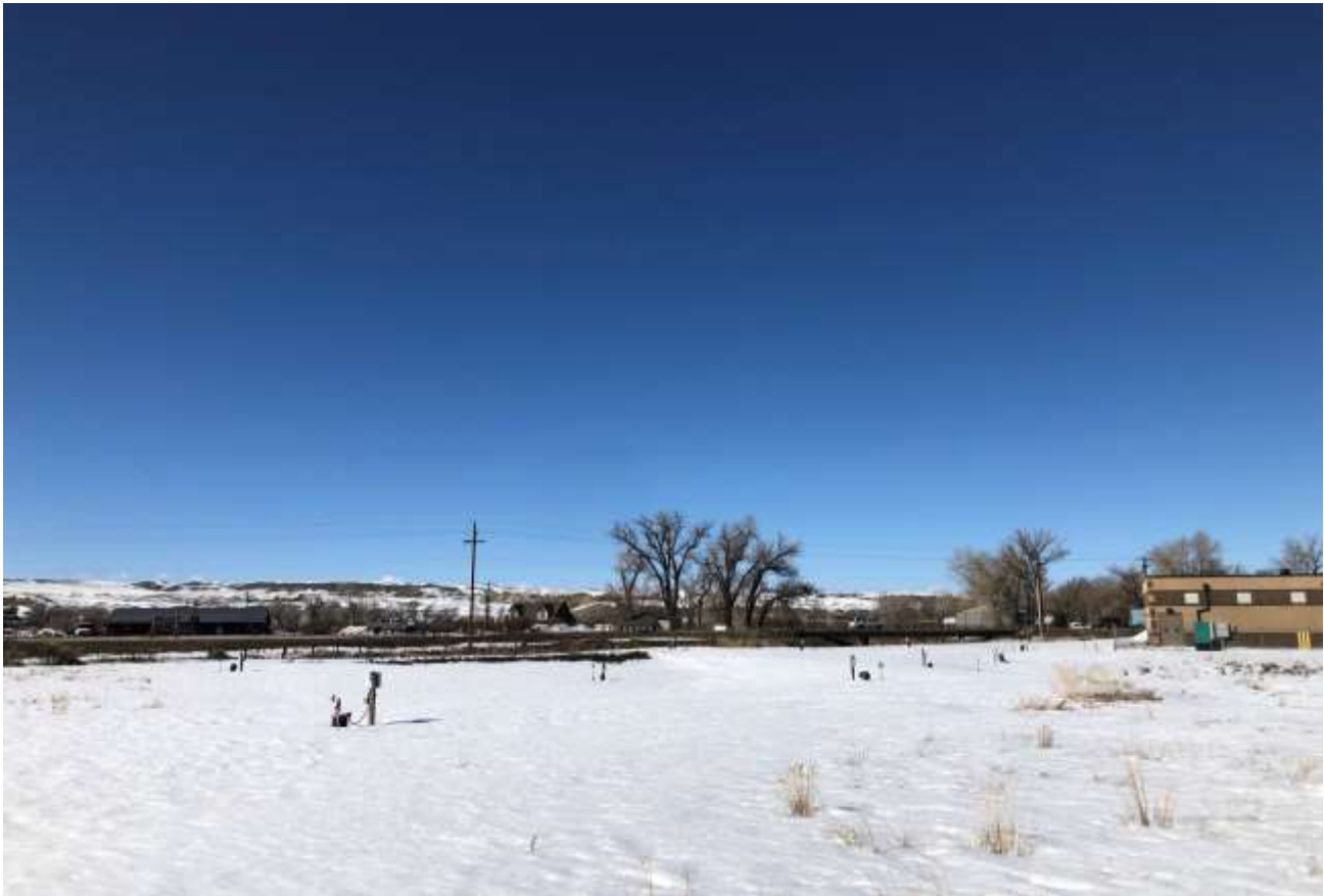
Alluvial Wellfield and Treatment Plant
