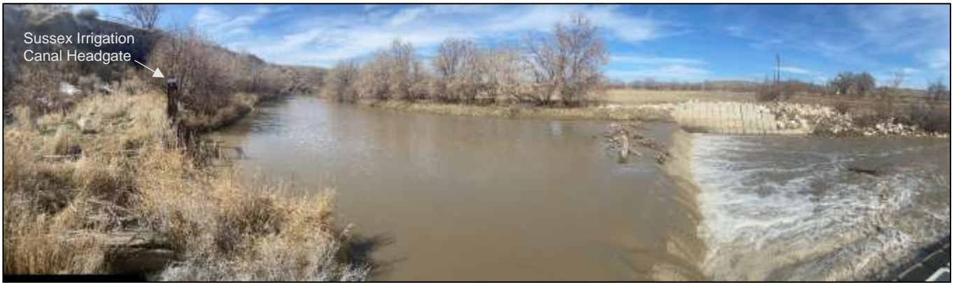
Middle Fork Powder River diversion dam and headgate (left) to Sussex Irrigation Canal. These structures were constructed in 1994 and are reported by the District be in good condition.
