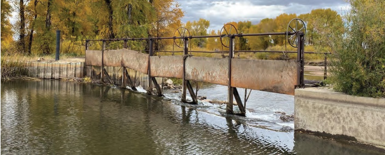
Dowlin Diversion viewed from upstream
