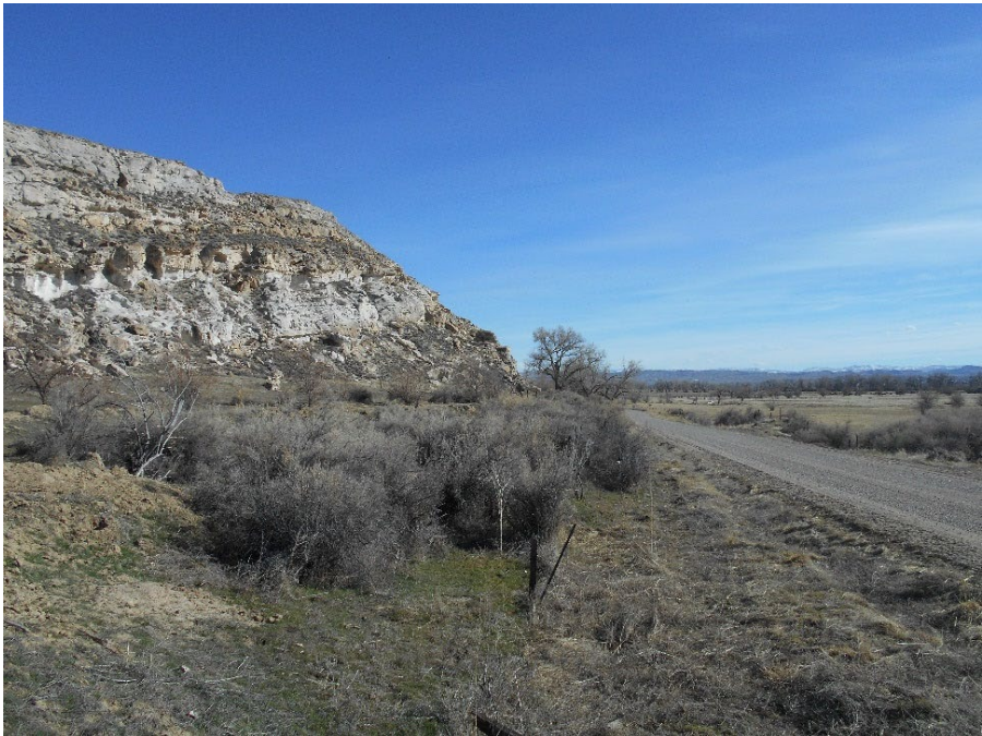
Kirby Ditch to the left under hillslope
