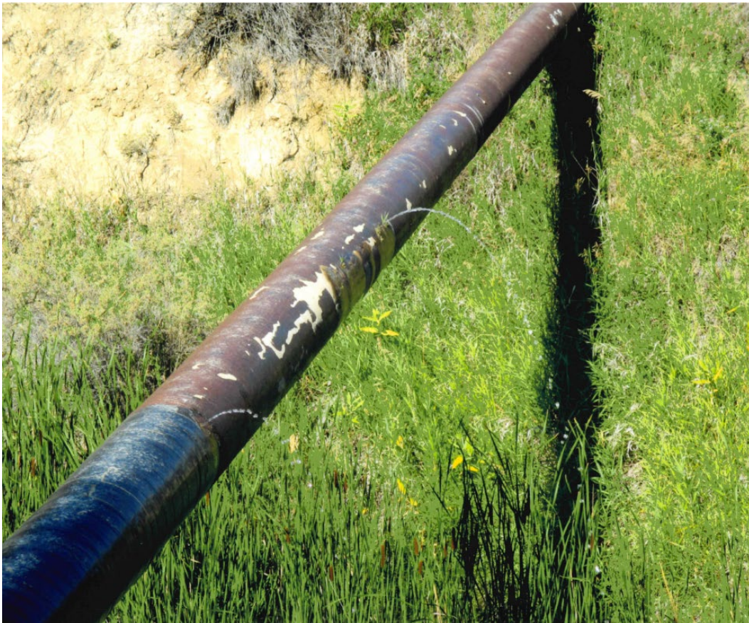
Piped Portion of D44-10
