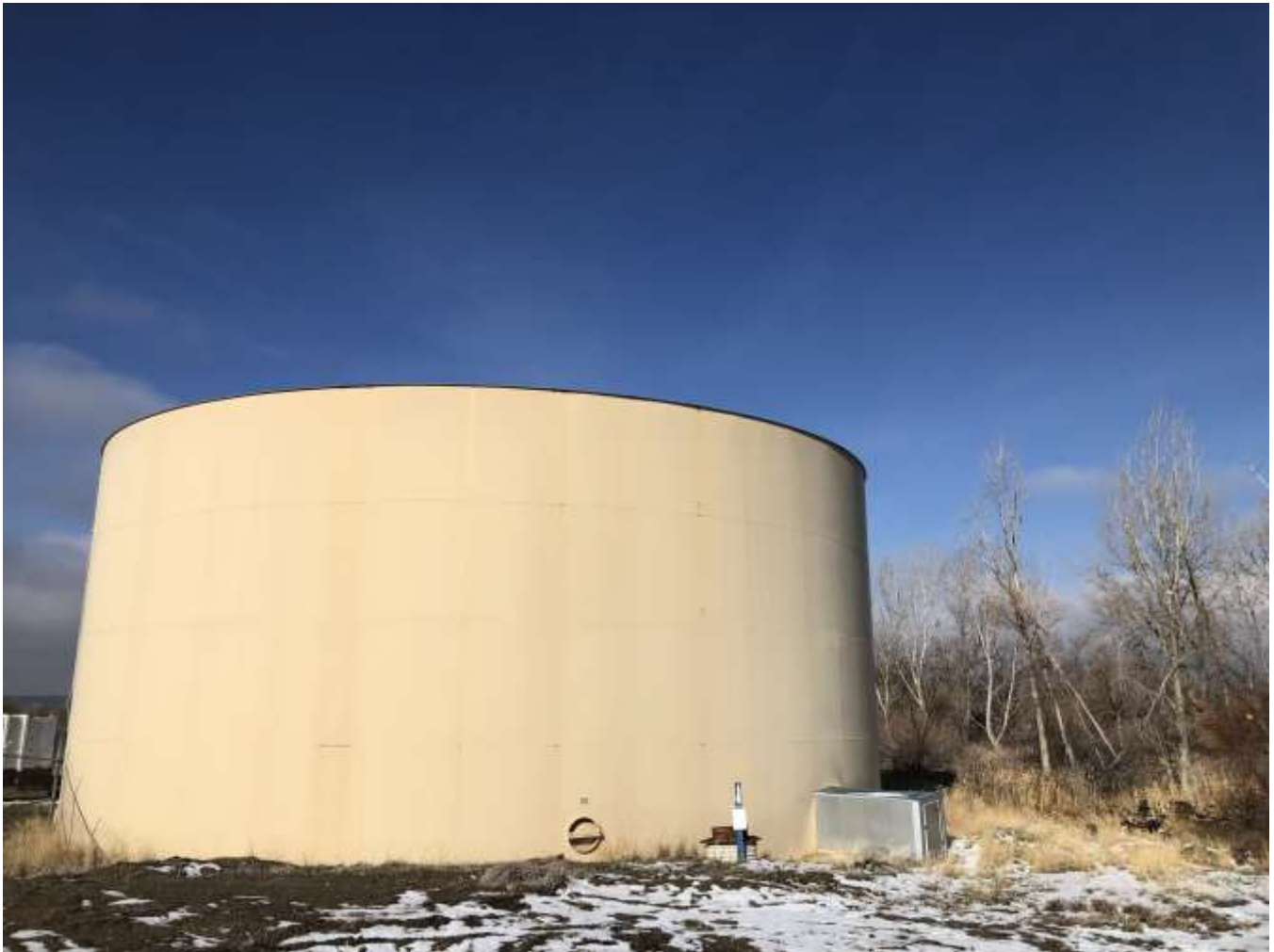
One Million Gallon Storage Tank
