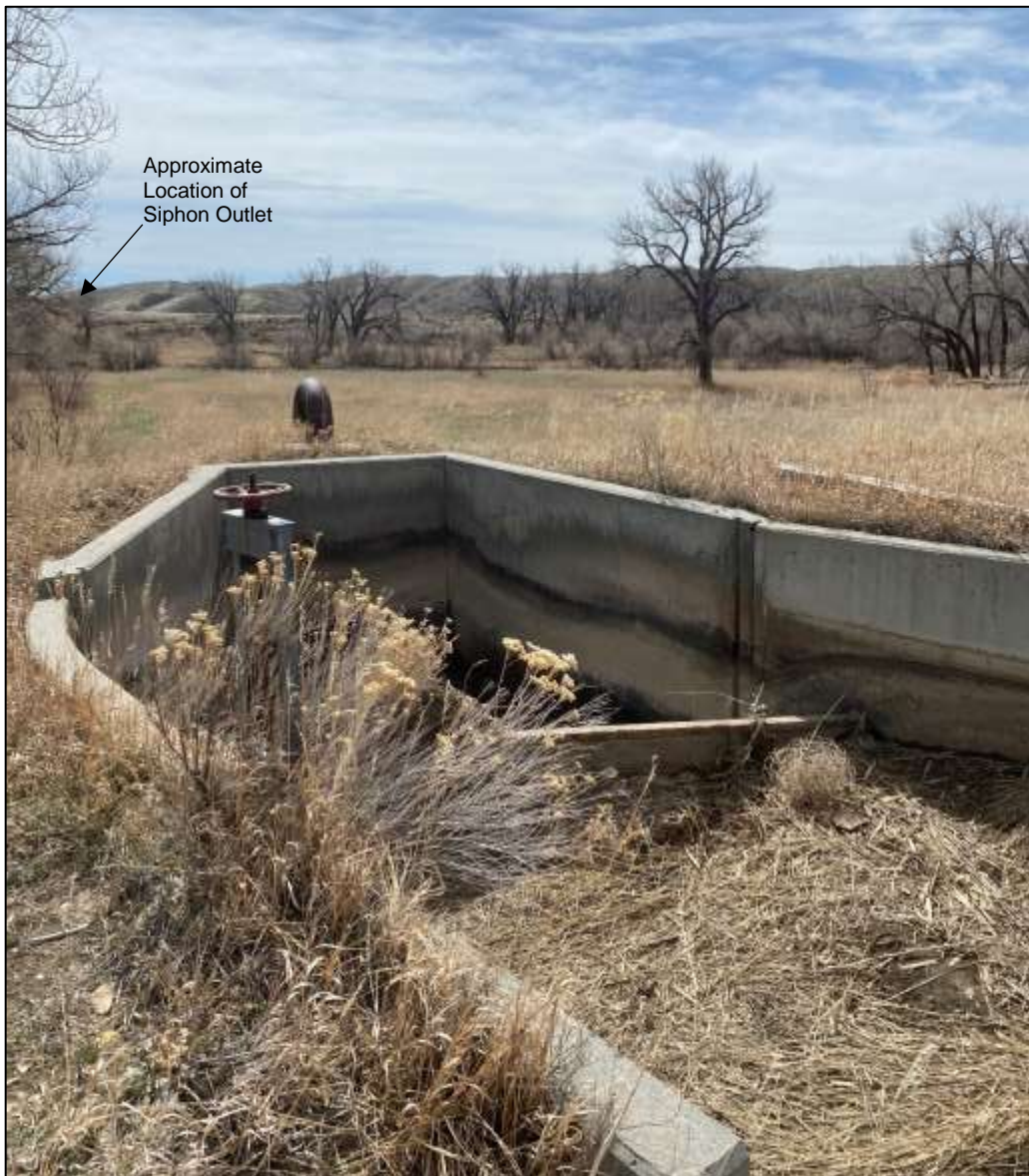
Siphon extending canal under South Fork Powder River was also constructed in 1994 and is reported to be in good condition. The Sussex Irrigation Canal has four siphons.
