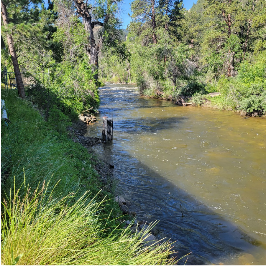
River Adjacent Infiltration Gallery
