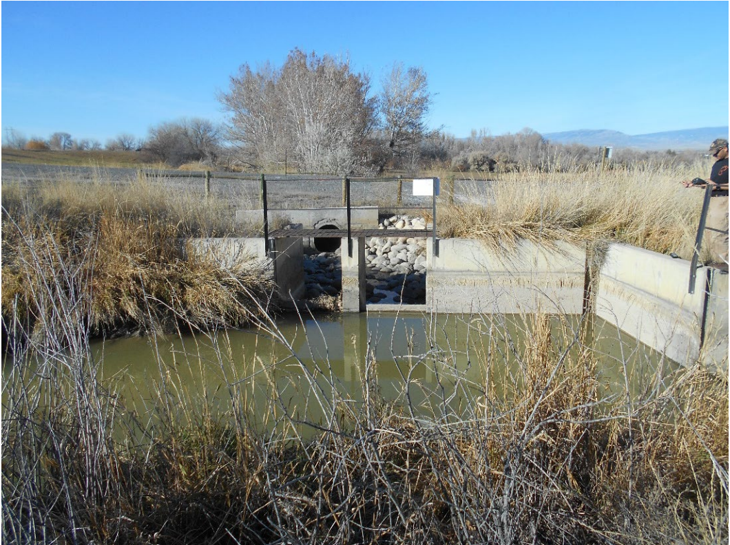
BENCH DIVERSION - BENCH STOP LOG WALL
