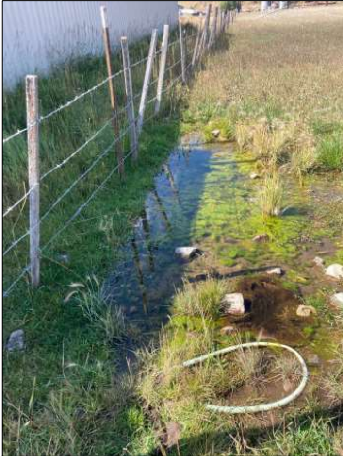
Examples of Leakage on Main Conveyance Pipeline. All repairs are completed by Upper Strawberry Canal Company.
