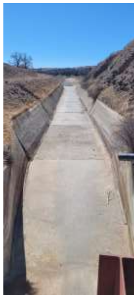
Measurement Flume (System Chokepoint)
