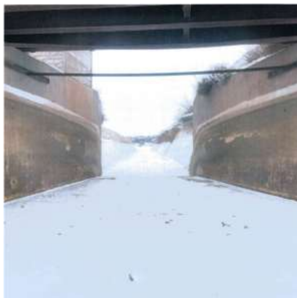
Measurement Flume (System Chokepoint)
