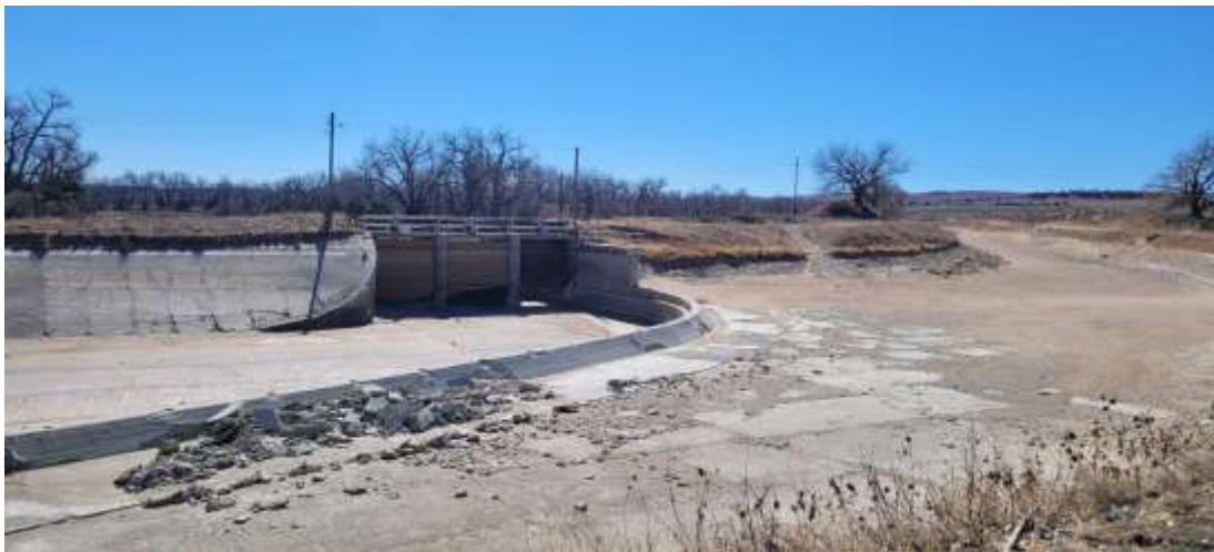
Silt Basin and Gates
