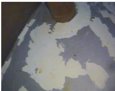
Interior Floor Patching
