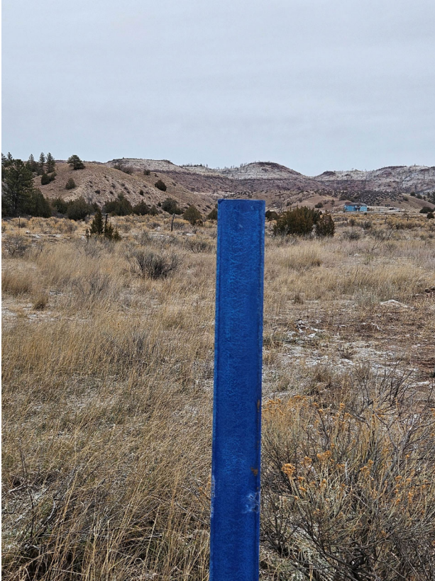
Hartville Transmission Line (Looking to Town)
