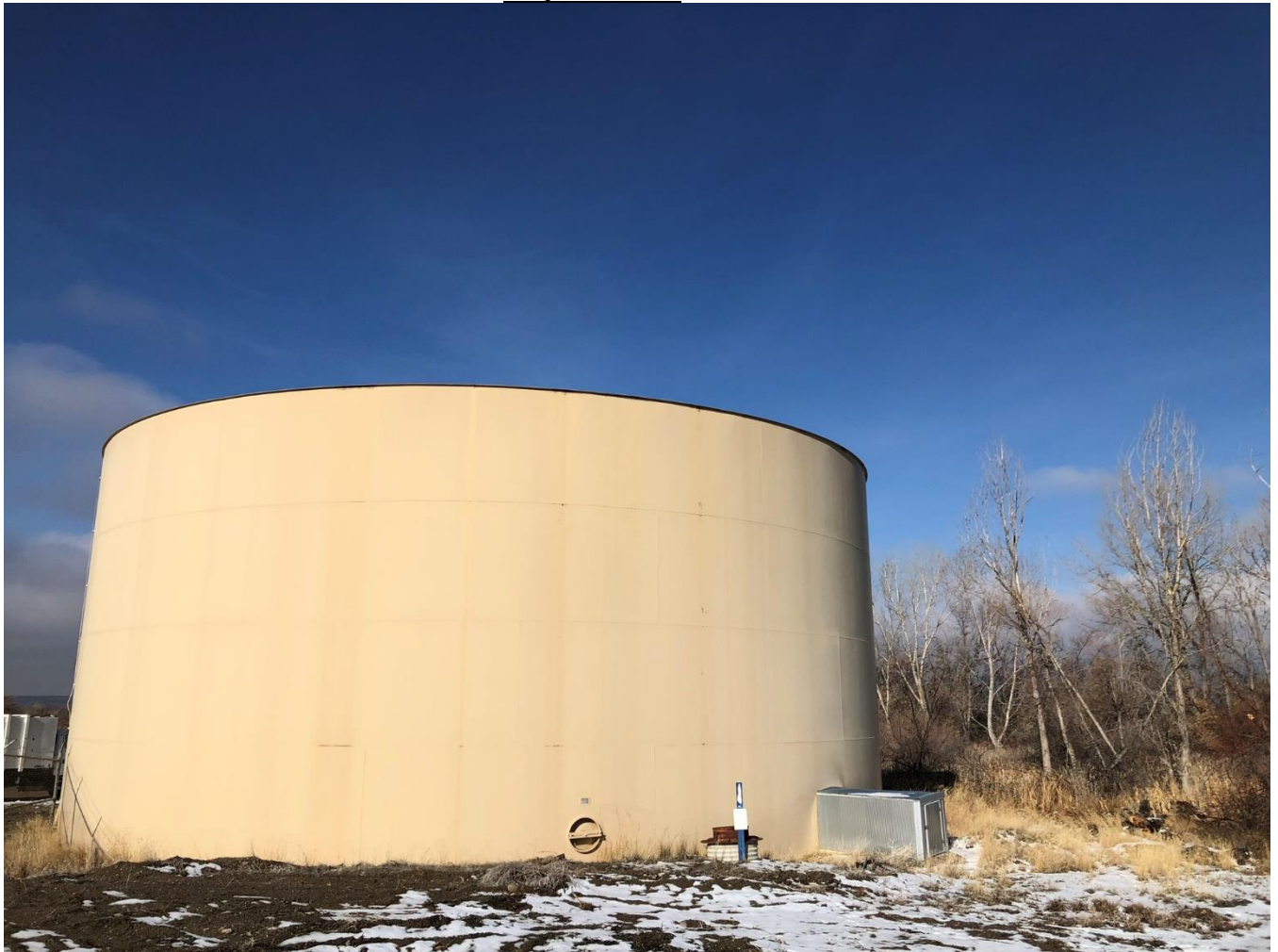
One Million Gallon Storage Tank
