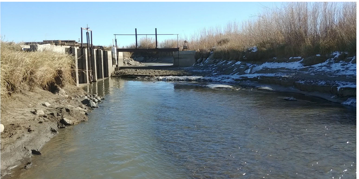
Diamond Creek Spill view of the canal (Water Out)
