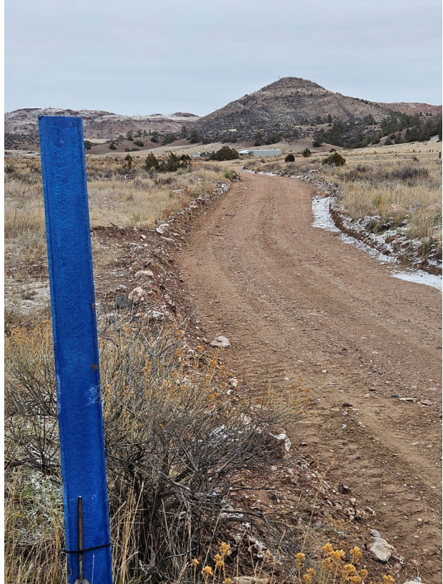
Hartville Transmission Line (Looking to Wells)
