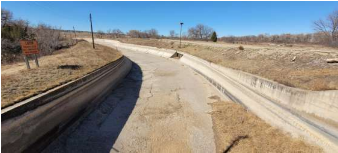
Chute Below Gates
