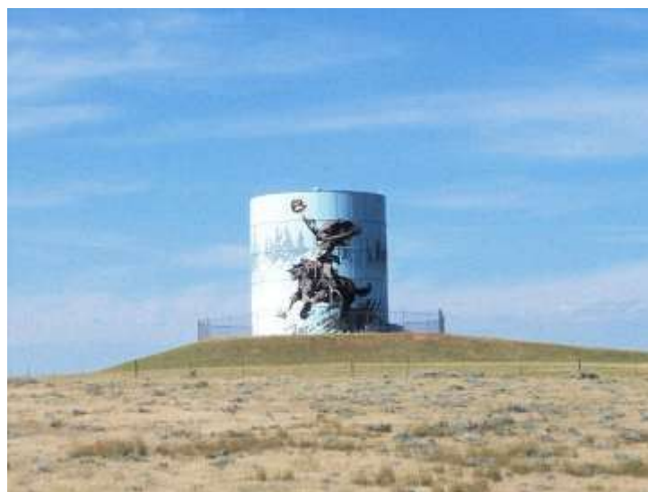
Sleepy Hollow Water Storage Tank at the end of Brom Street.
