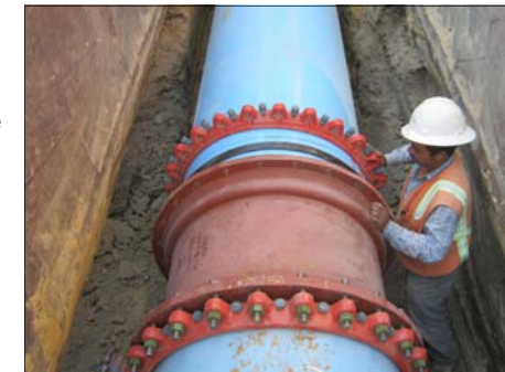
Highway 50 Waterline Project
