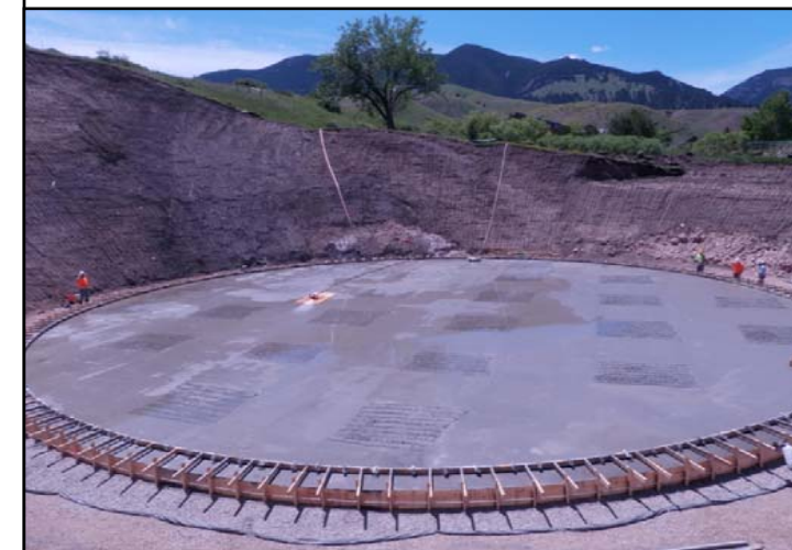
Tank Concrete Foundation
