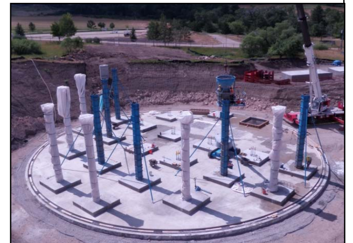
Tank Roof Support Columns
