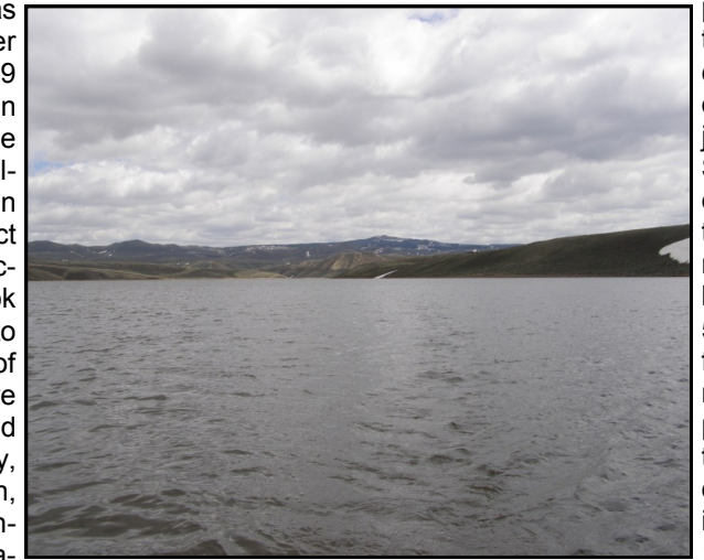
High Savery Dam and Reservoir
